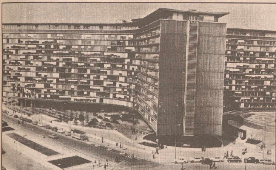
Trollhulen i Brussel (foto Nordlys).
